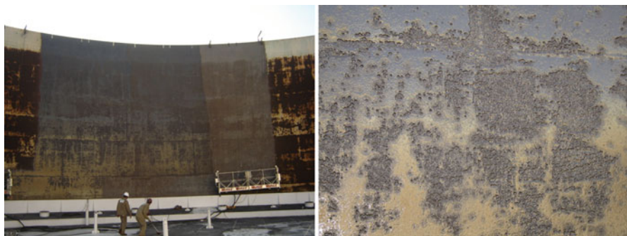
Fig. 9 Defects found in steel tank: inside view ( left ) and corroded surface detail ( right )
