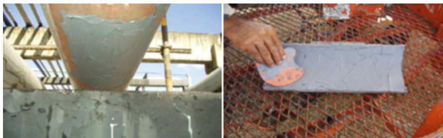
Fig. 13 Adhesive application: over pipe surface ( left ) and the saddle ( right )
