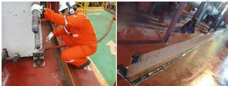
Fig. 14 Coaming: around an equipment ( left ) and detail of welded coaming ( right )
