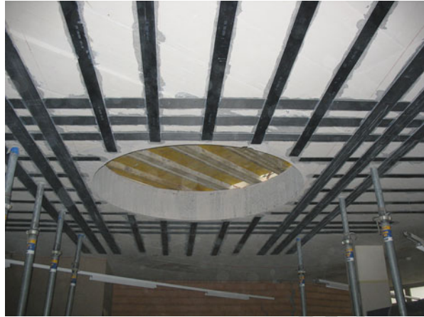
Fig. 3 Ceiling strengthened with CFRP plates (Source: Stahlton AG)
