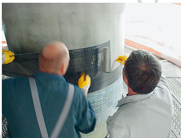
Fig. 5 Strengthening of a column by a direct laminating approach (Source: StoCretec GmbH)
