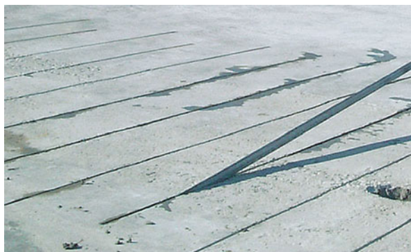
Fig. 4 Strengthened concrete structure achieved by bonding CFRP strips into slots (Source: StoCretec GmbH)
