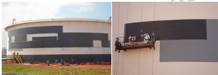
Fig. 10 Repairing a storage tank: repair overview ( left ) and repair application ( right )
